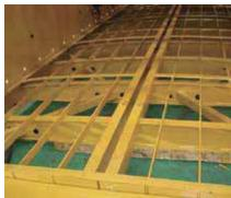
Standard Cambered deck frames. are strengthened with herringbone bracing on each end.
